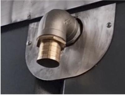
13- There is a outlet connection from the bath to pressure unit that you can use in case of inlet water to pressure unit. [Out to Pressure Unit]
